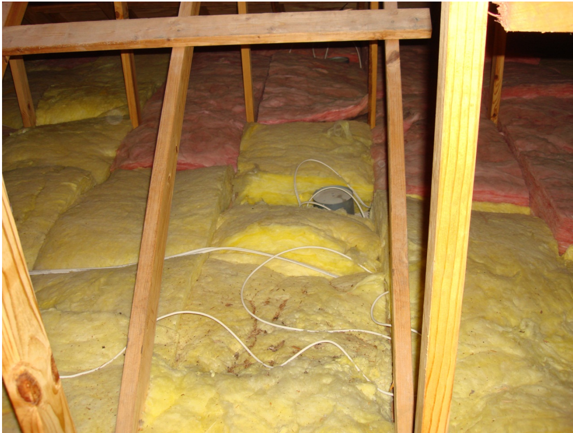
Hole in attic insulation for recessed light
