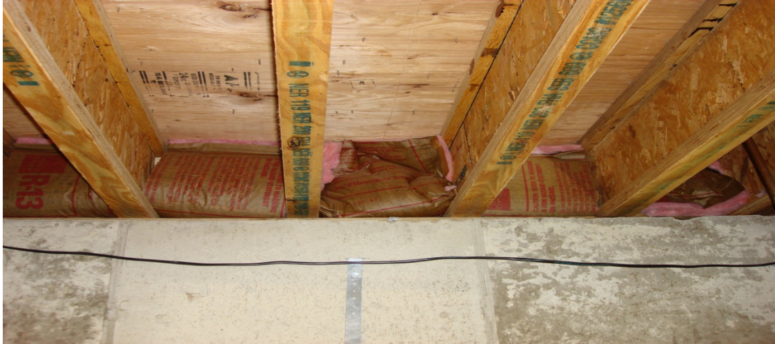
Basement rim Joist insulation
