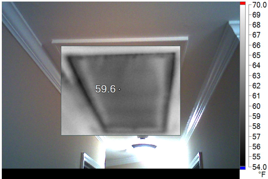
Thermal and air leak at attic hatch
